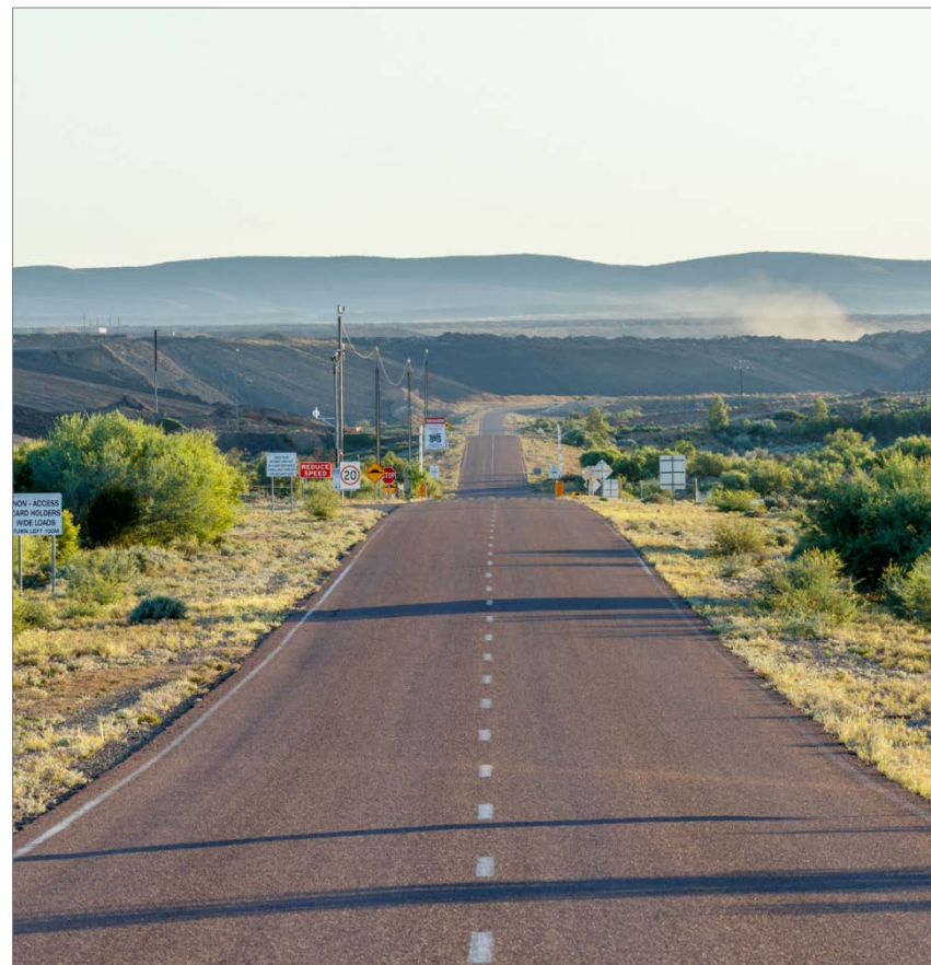
Entrance to Leigh Creek site
