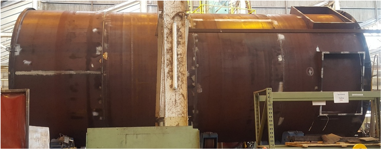
Thermal Oxidiser casing fabrication nearing completion
