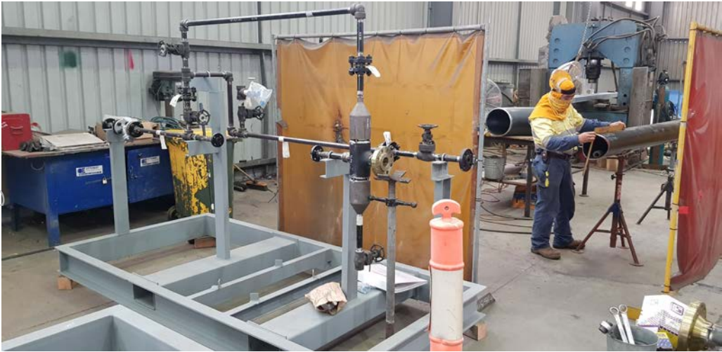
Module fabrication assembly underway
